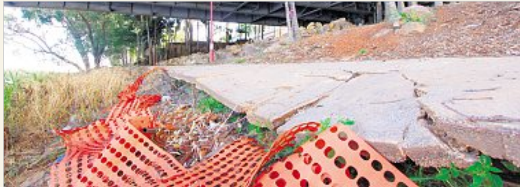
BEING REPLACED: Work starts next week on repairing the flood-damaged path under the Fitzroy Bridge. PHOTO: CHRIS ISON ROK130613CPATH2
